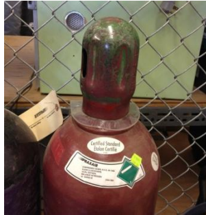
Figure 9: Cylinder cap. Image courtesy of WSEP.
